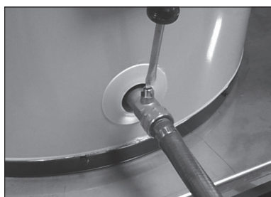
Draining the old water heater.
