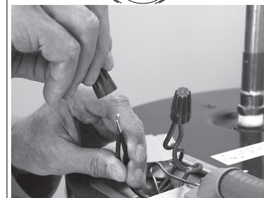
Connecting the electrical wires.
