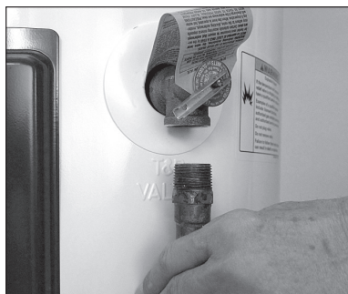
Removing the T&P Relief Valve discharge pipe.
